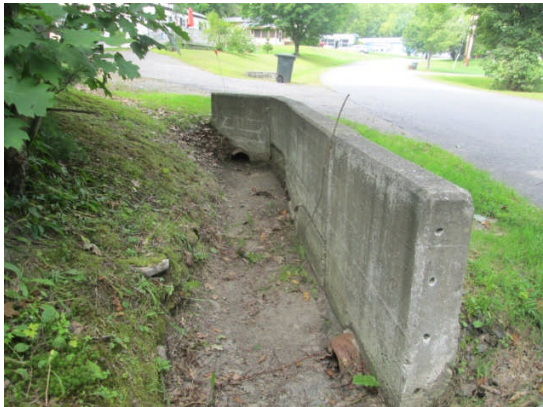
blocked drainage pipe
