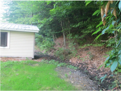
Drainage swale base of hill
