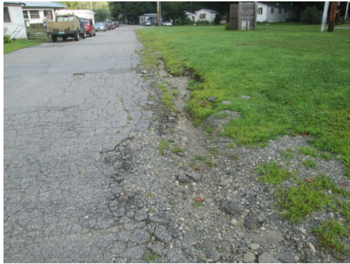
improper road drainage, wash out 1
