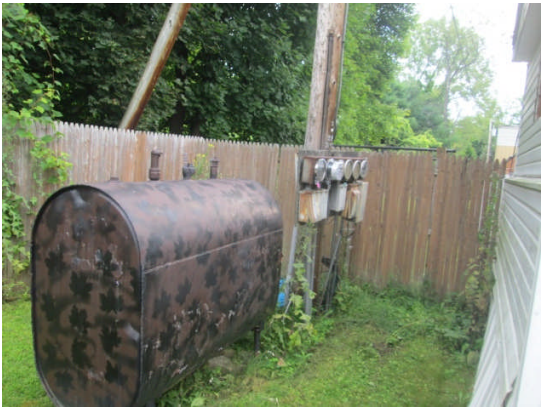
marginal corrosion on tank
