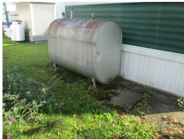
corrosion on tank, fair condition
