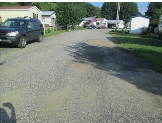
Deteriorated asphalt
