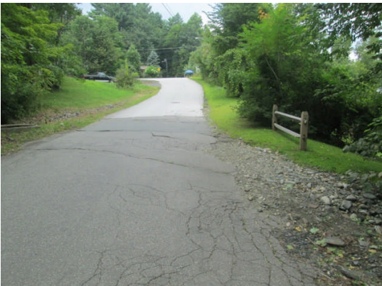
Areas of improper drainage
