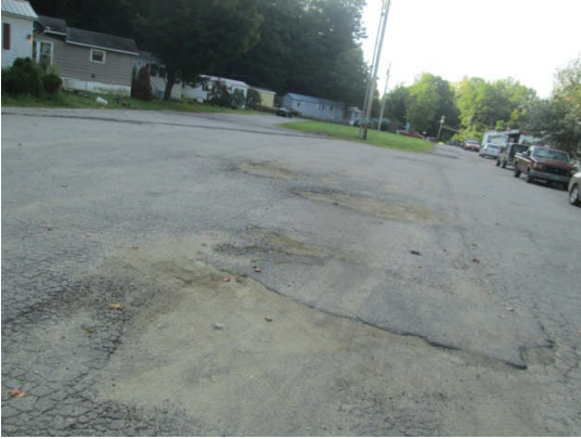
Deteriorated road surface
